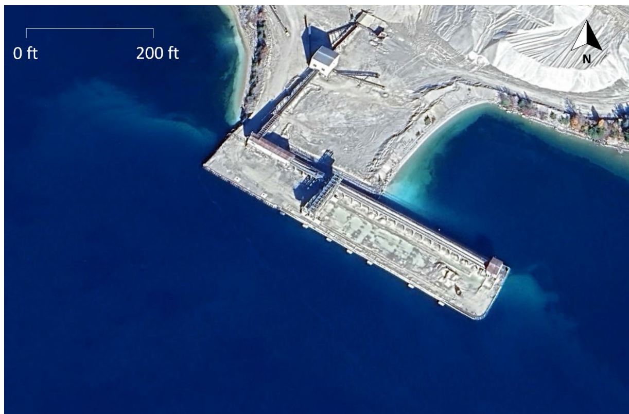
Figure 4. The Cedarville dock in Port Dolomite, Michigan. (Background source: Google Earth)
